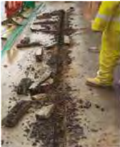
Fig. 2.1.2 Manual Narrow trenching
