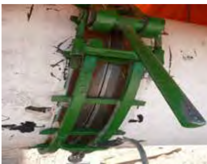
2.4.10 Pipe Fitup with External Clamp
