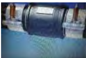
Fig. 2.6.37 Pipe and socket full assembly
