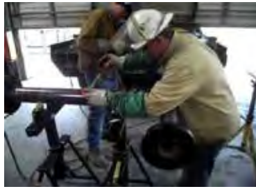
Fig. 1.7.40 Pipe to Tee Fitup and Alignment
