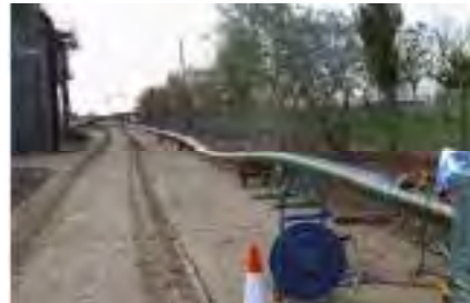
Fig. 2.6.28 Stringed PE pipe ready for lowering
