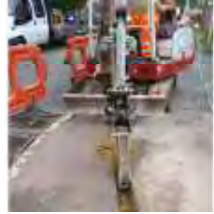
Fig. 2.1.11 Narrow trenching with modified excavator buckets
