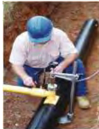
Fig 2.6.71 Saddle electrofusion arrangement
