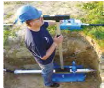
Fig. 2.1.21 Impact moling monitoring
