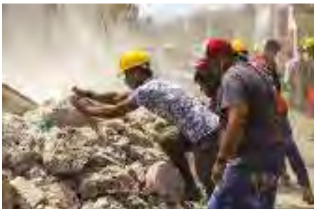
Fig. 4.4.14 Response at Construction side
