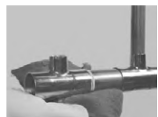
Fig. 2.3.152 Clean off Flux Residue
