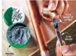
Fig. 1.8.124 Fluxing of Tubes
