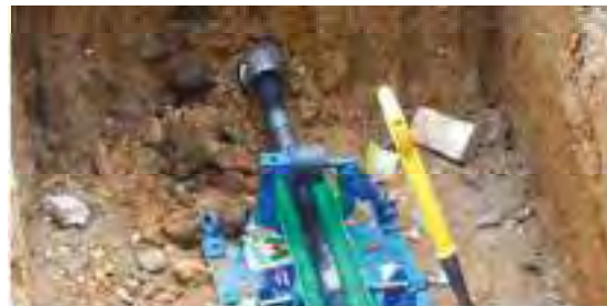
Fig. 2.1.17 Impact moling hammer in its launch pit
