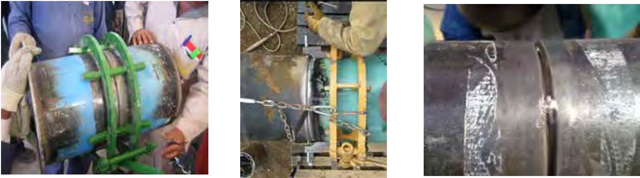
Fig. 1.7.34 Pipe Fitup and Alignment
