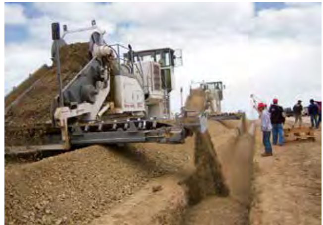
2.4.28 Pipeline Trench Back Filling
