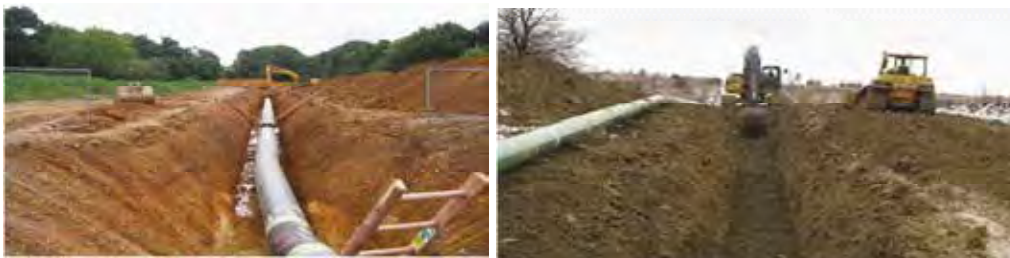
Fig. 2.1.1 Conventional trenching for pipeline installation– bedding& laying
