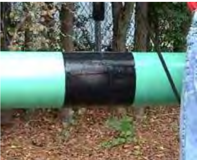
2.4.23 Weld Joint Coating (Shrink Sleeve)
