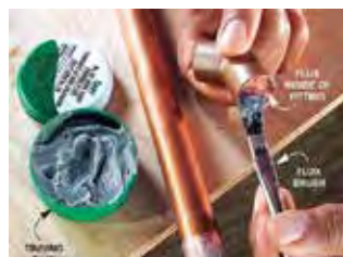
Fig. 2.3.150 Fluxing of Tubes
