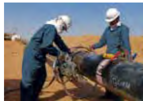
2.4.19 Automatic Ultrasonic Testing
