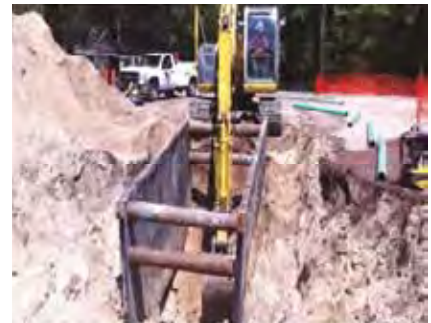
Fig. 4.1.41 Pipeline trench box
