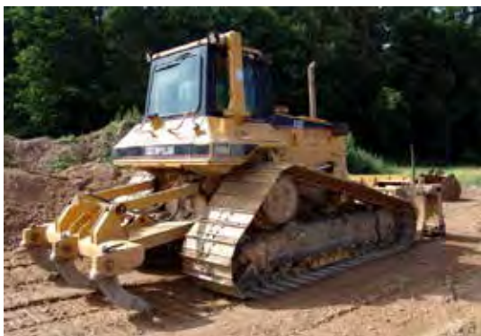
2.4.2. Pipeline Route Grading
