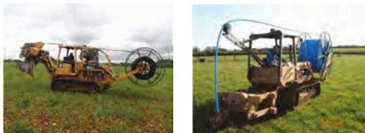
Fig. 2.1.12 Mole ploughing equipment in the field
