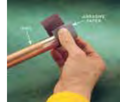
Fig. 1.8.122 Cleaning of Tube Ends
