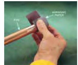
Fig. 2.3.148 Cleaning of Tube Ends
