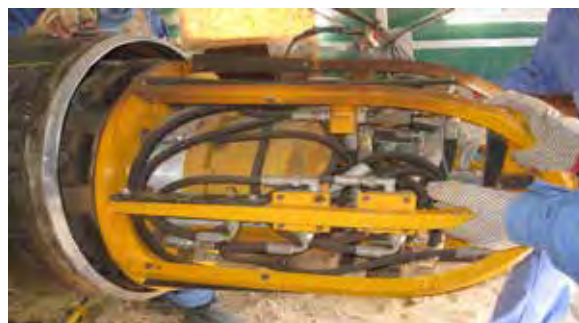
2.4.11 Pipe Fitup with Internal Clamp
