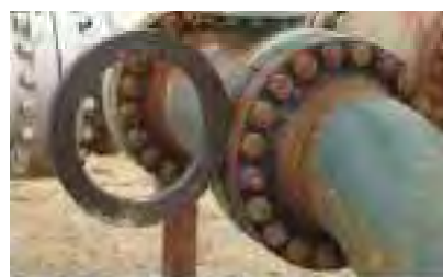
Fig. 1.5.13 Spectacle blind flange – closed
