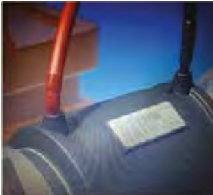
Fig. 2.6.42 Connecting leads to fitting
