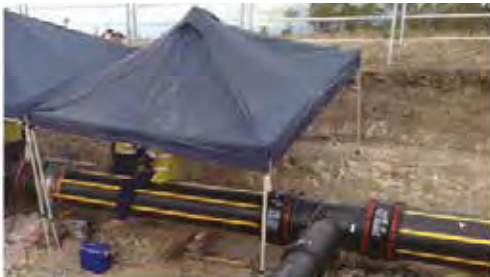
Fig. 2.6.27 typical tent during PE pipe joining
