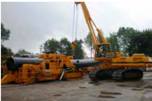
2.4.6 Pipe Cold Bend
