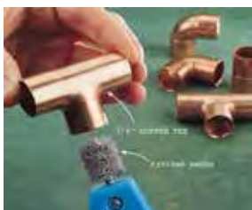
Fig. 2.3.149 Cleaning of Fitting
