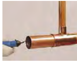
Fig. 1.8.121 Deburring of Tube Ends
