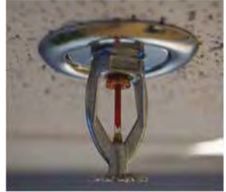
Fig. 4.2.12 Water sprinkling system
