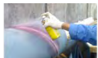
2.4.21 Liquid Penetrant Testing
