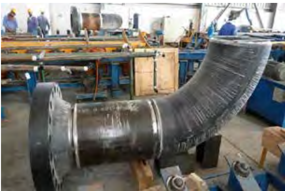
Fig. 1.7.36 Pipe to Elbow Fitup and Alignment
