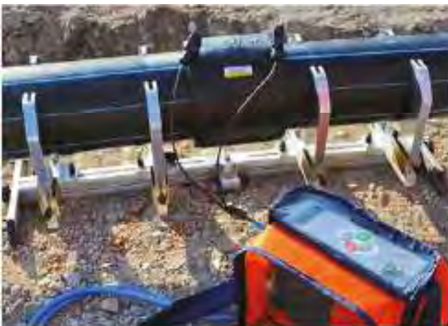
Fig. 2.6.39 Electrofusion arrangement
