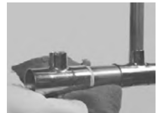
Fig. 1.8.126 Clean off Flux Residue
