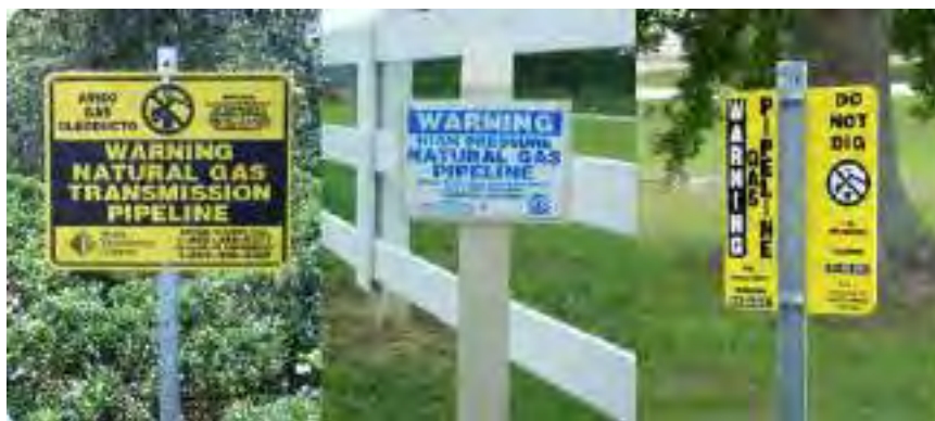
2.4.33 Marker Post Installation (Pipeline)
