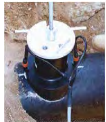
Fig. 2.6.87 Fusion arrangement
