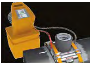
Fig. 2.6.77 Performing fusion welding
