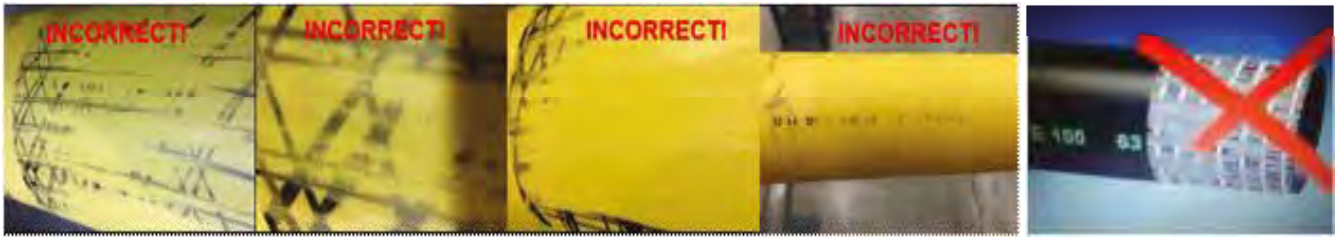
Fig. 2.4.16 Incorrect scraping
