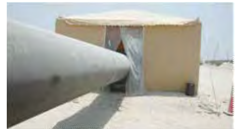
Fig. 2.4.22 Protecting fusion area with tent
