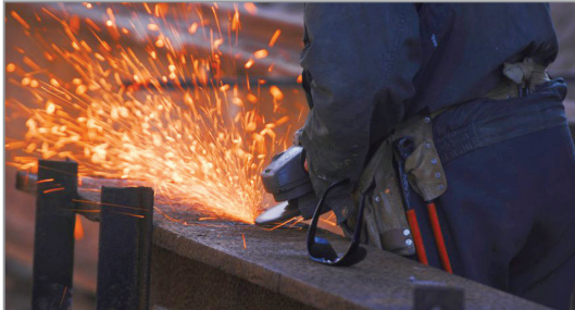
Fig. 2.1.5. LPG use at construction site
