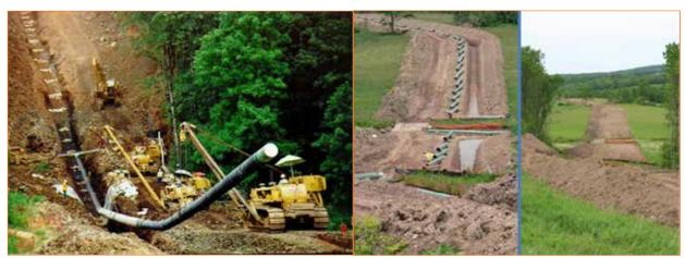
Fig: 2.1.15 Lowering pipe into the trench
