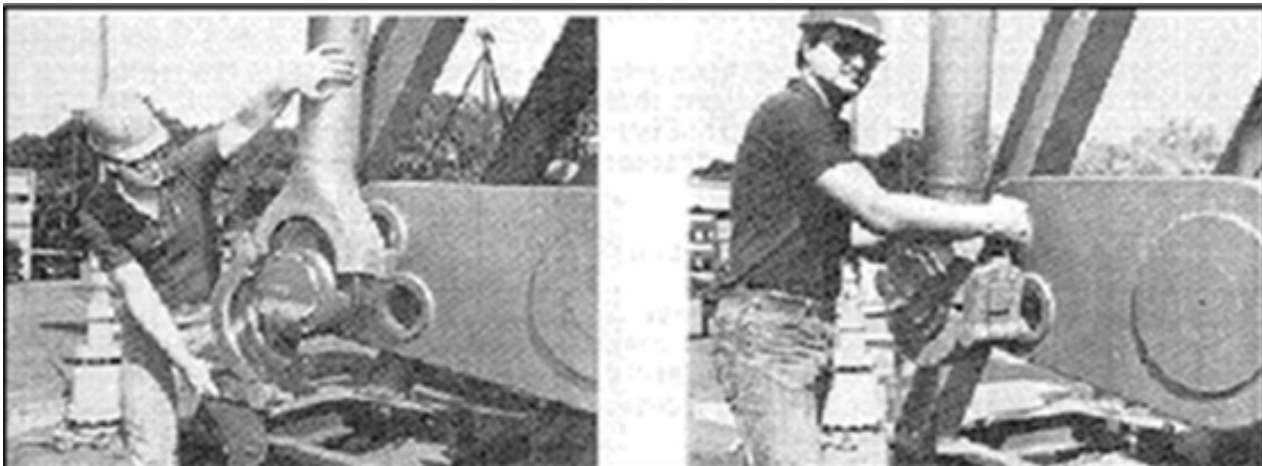
Figure 2.3.8: Workers at site inspecting the equipment
