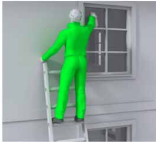
Figure 3.2.7: Following 3 point contact and not overreaching the work area
