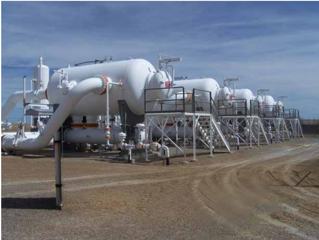
Figure 2.3.1 Coalescer machines to separate oil and water from the emulsion
