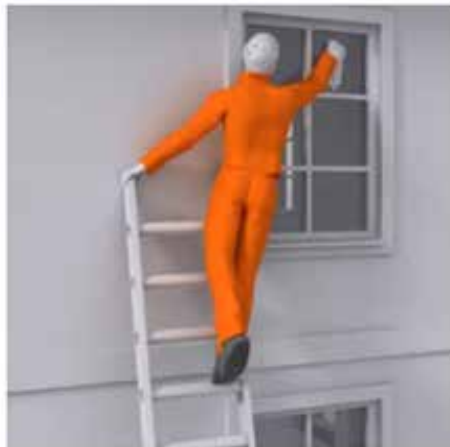
Figure 3.2.6: Not following 3 point contact and overreaching an area
