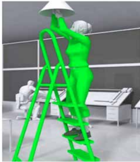
Figure 3.2.4: Ensuring that both the legs are on the same platform (step) with the knees supported to the stepladder and availability of handhold
