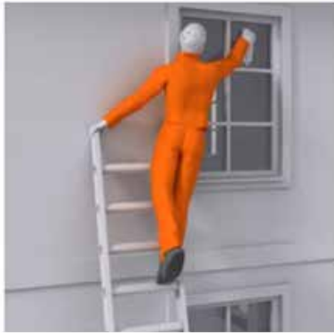
Figure 3.5.6: Not following 3 point contact and overreaching an area
