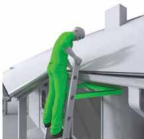
Figure 3.5.5: Taking the help of stand-off devices to get a strong resting point.
