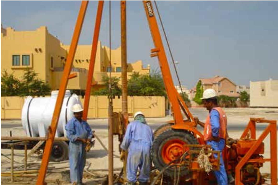
Figure 2.2.10: Percussion or Cable Drilling Technique
