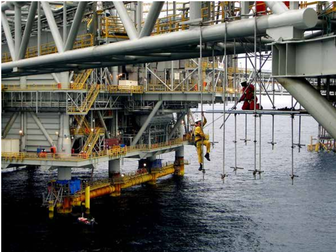
Picture 2.2.1: Working at Height
