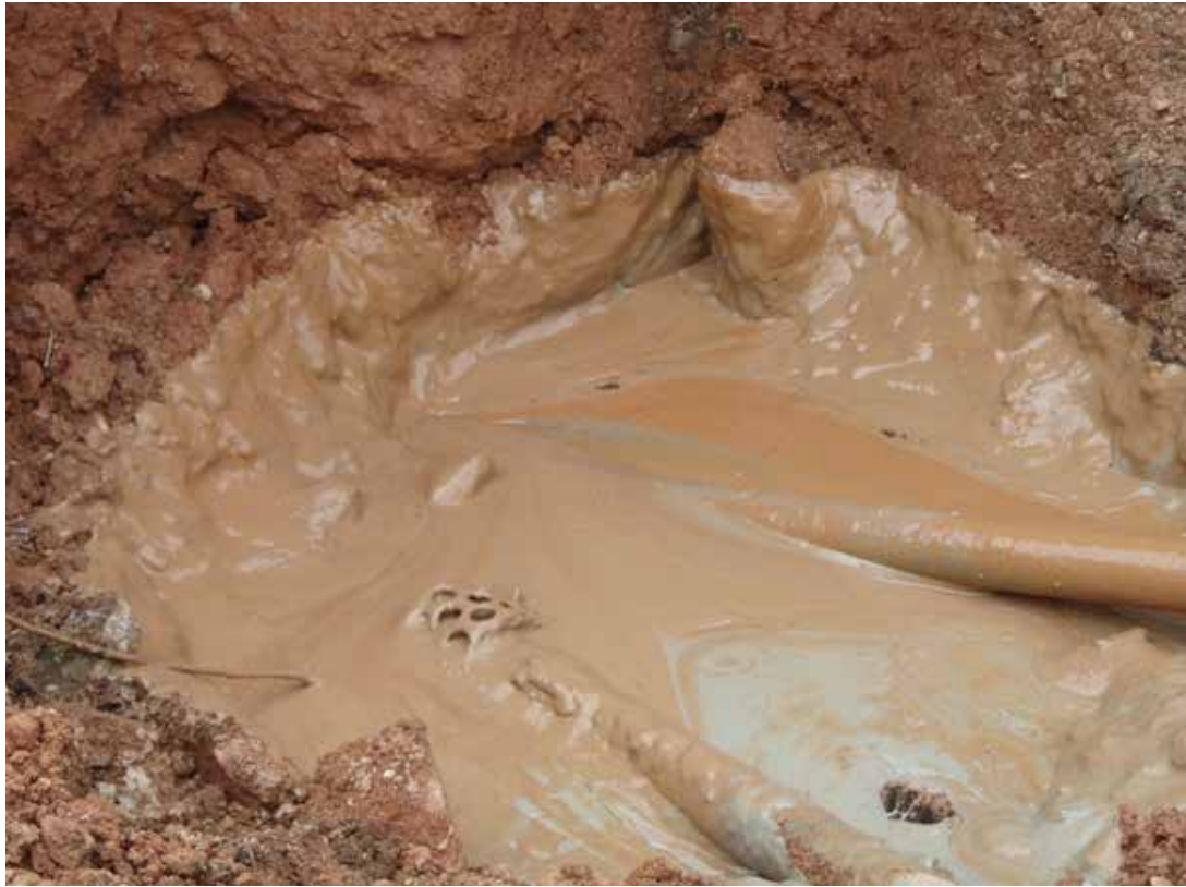
Figure 2.2.14: Horizontal Well Drilling Mud Pit
