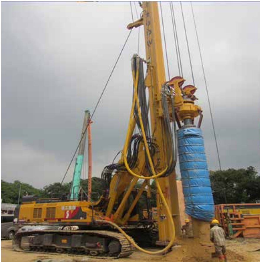
Figure 2.2.12.: Rotary Percussion Drilling
