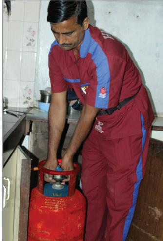
Fig 2.3.8 Fit the pressure regulator
