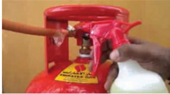
Fig. 3.1.7. Check LPG leakage with soap solution
