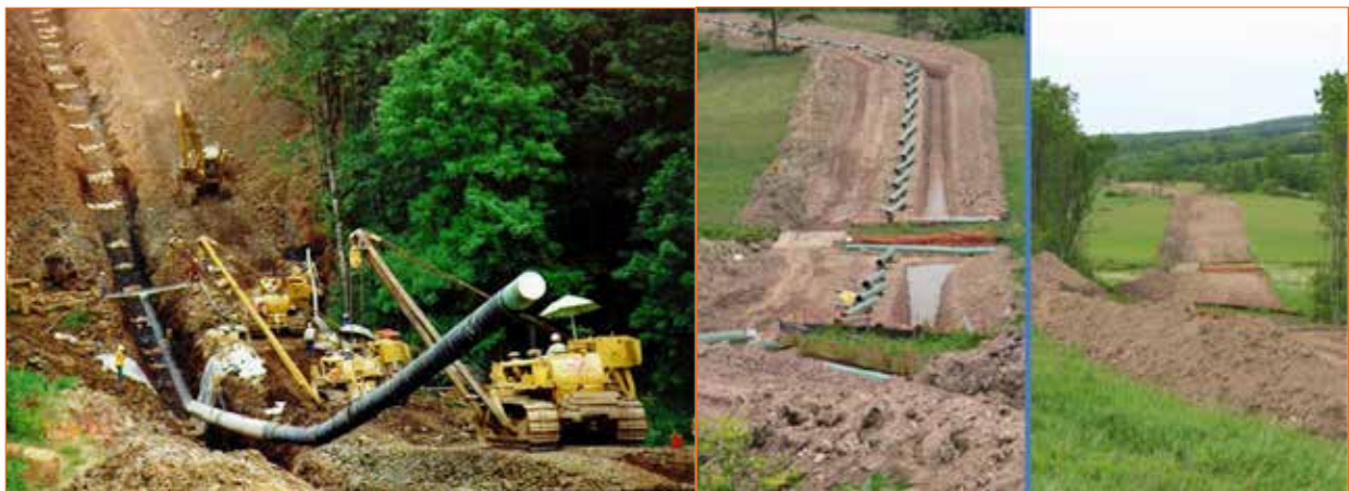
Fig: 2.1.15 Lowering pipe into the trench
