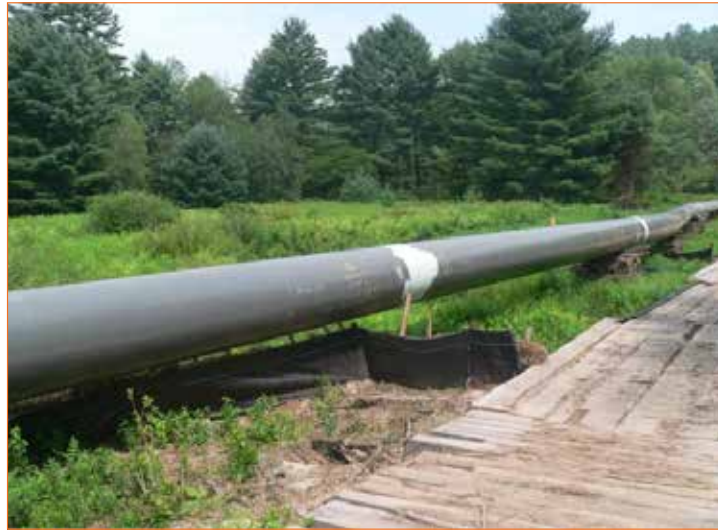
Fig: 2.1.14 Pipe ready to be placed underground after contouring and welding.
